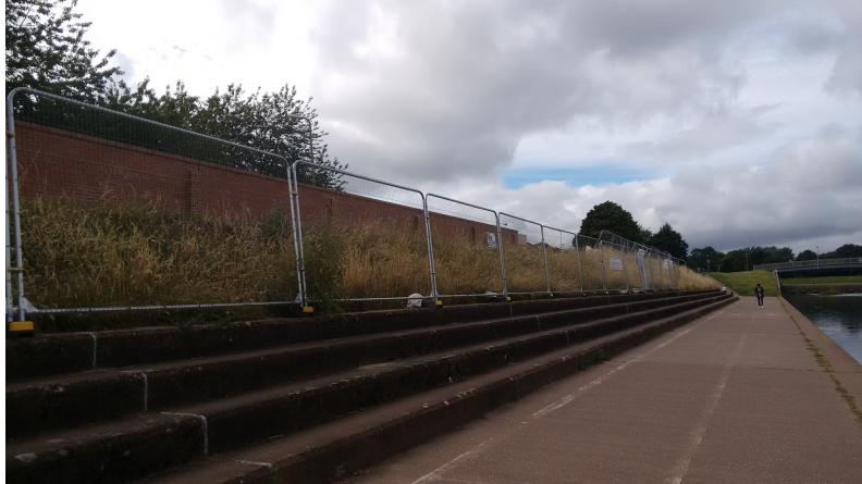
Figure 6.3: Construction of a new wall that will prevent flooding of houses and businesses in a 100 year storm in the St. Thomas area of Exeter. (Source: the author).
