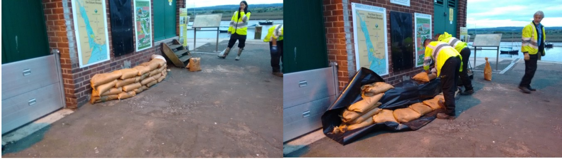
Figure 6.9: A demonstration of the mounting of sandbags by the EA and the Fire Brigade at the Topsham community flood simulation exercise in September 2015. (Source: author)
