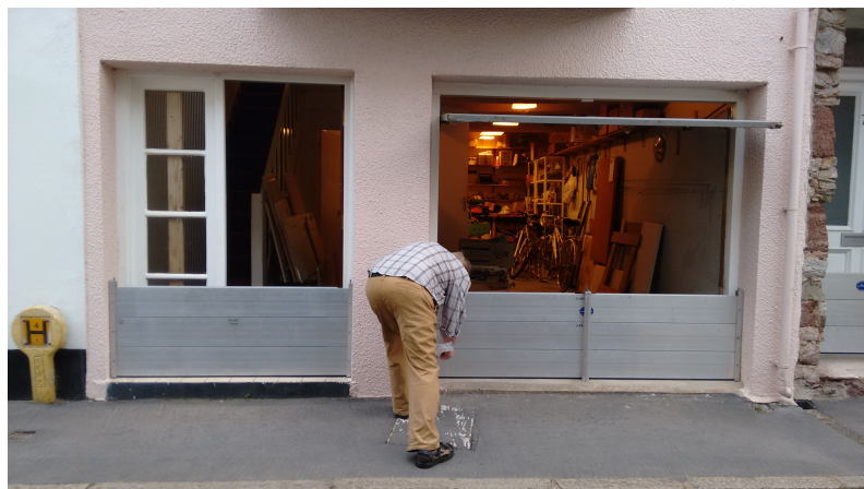
Figure 6.1: Topsham resident installing flood boards during community flood simulation activity (September 2015) (Source: the author).
