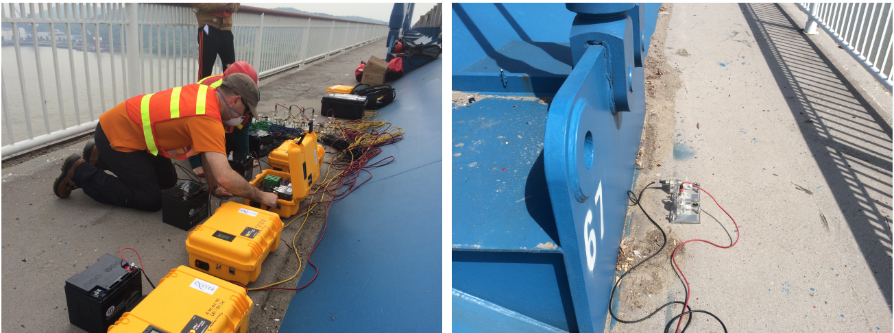
532 Figure 14: Setting up acquisition for initial huddle test and reference accelerometers at H67.
