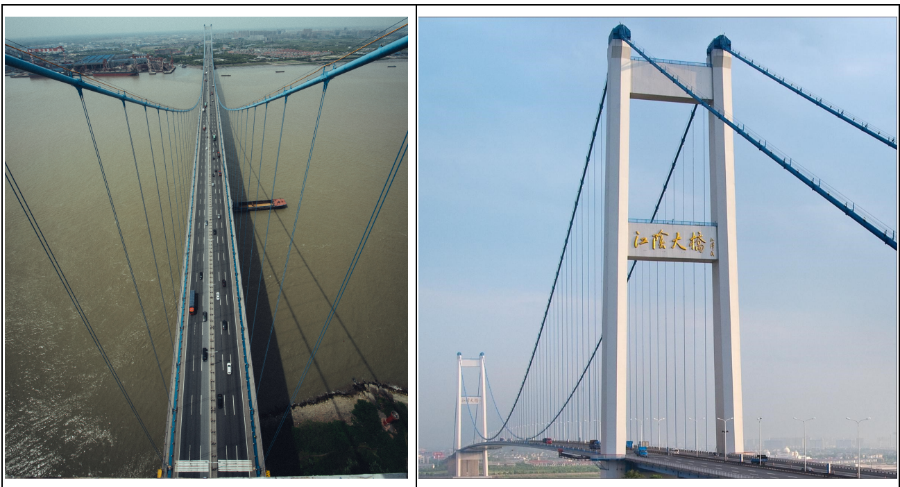
203 Figure 2: Jiangyin Bridge
