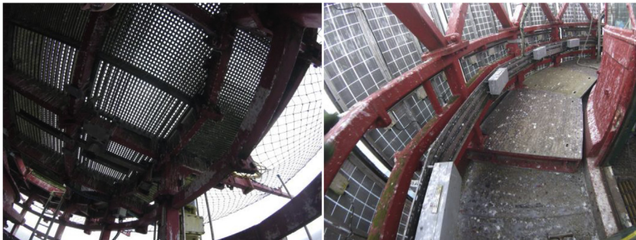
Fig. 17. Eddystone helideck views. Left: helipad, right: vertical structure rising from the gallery, with solar panels attached.
