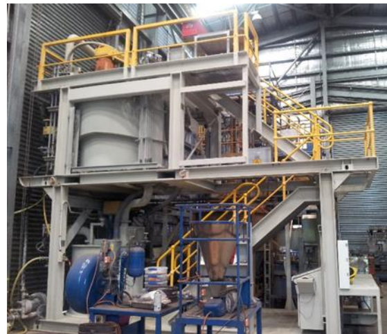
(b) On site side view
