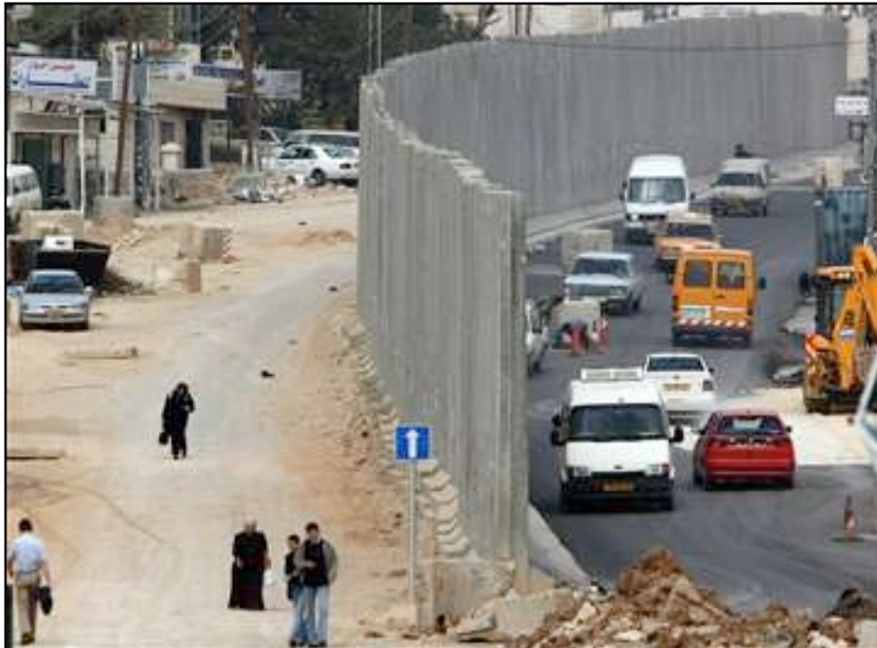
The Wall under construction in al-Ram, East Jerusalem 2006. Photo Credit: (B'Tselem 2017).
