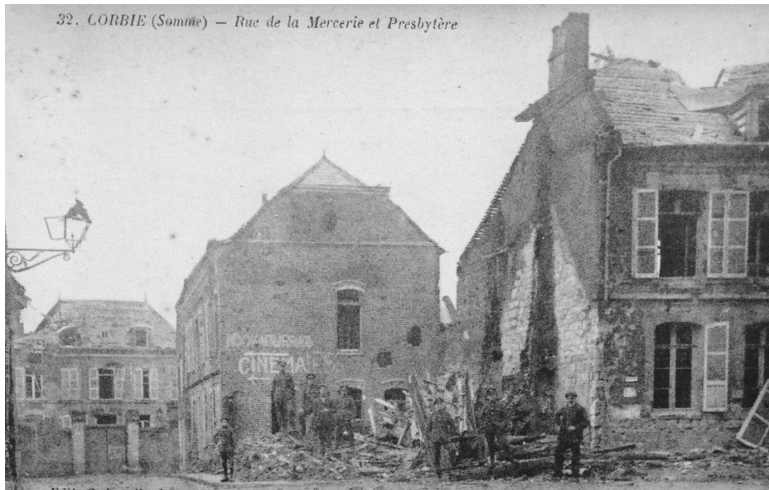
Fig. 2.9: Postcard showing a Cinema housed in a dilapidated building. Courtesy of the Nicholas Hiley Collection.
