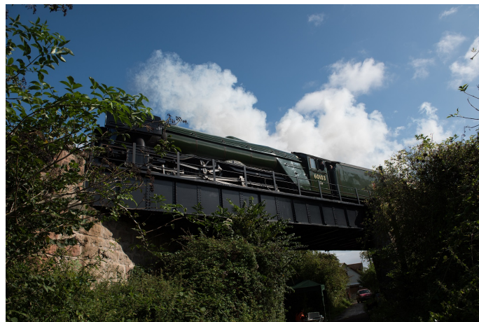
Figure 1: Flying Scotsman locomotive passing over the Mineral Line bridge
