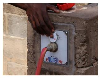
Figure 1. e-Tap and token in contact releasing water.
