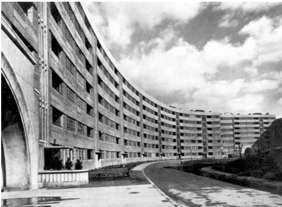
Fig. 4 Quarry Hill Flats, Oastler House, 1939
