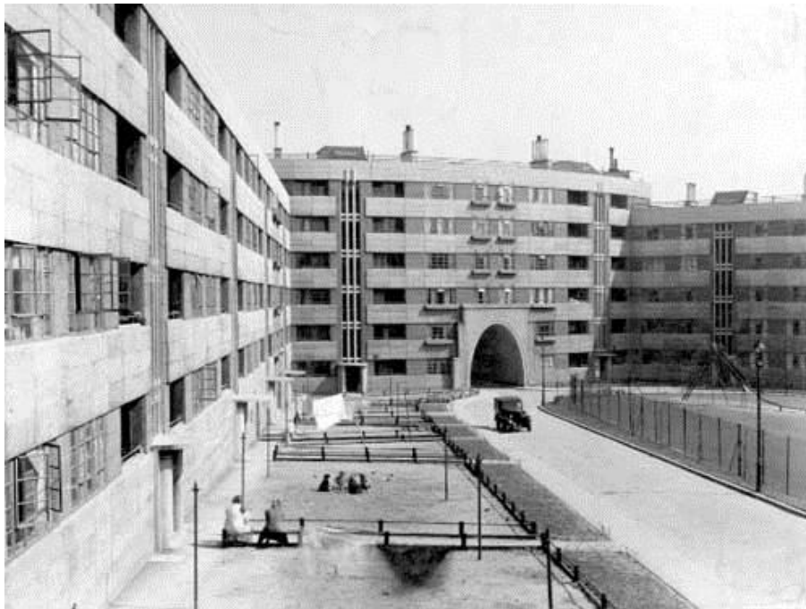
Fig. 6 Quarry Hill Flats, Lupton House, 1939
