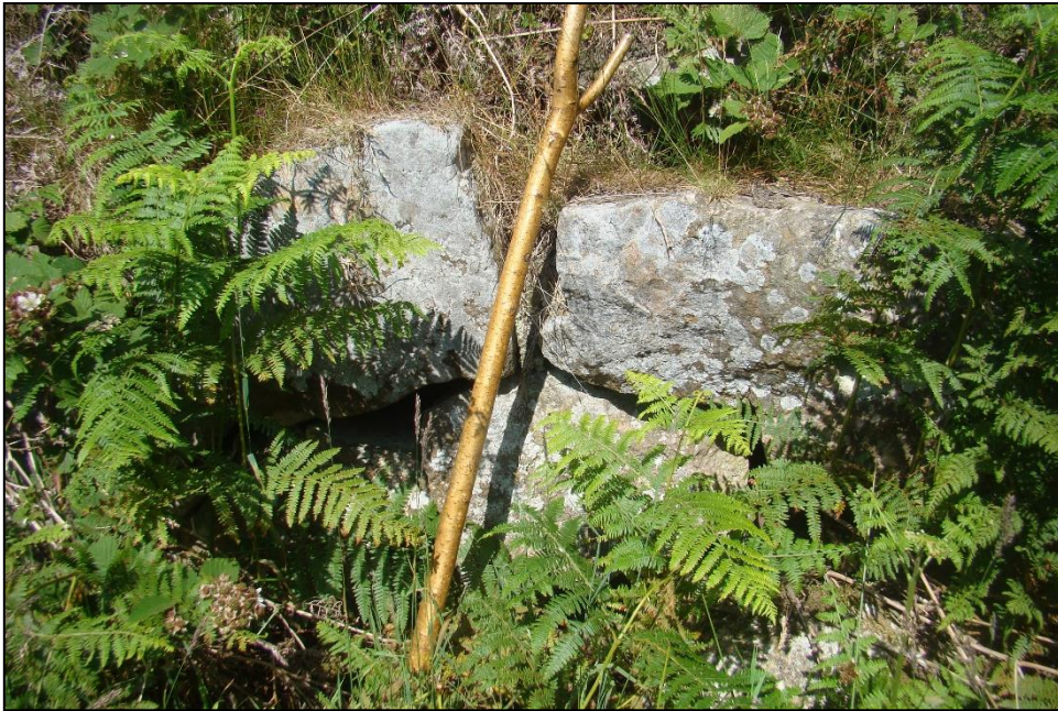
Figure 7: Revetment stone on bank of trackway beside Llanderfel chapel (Source: author).
