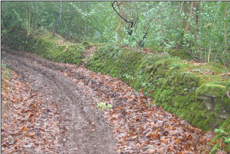
Figure 15: Further section of revetment wall (Source: author).
