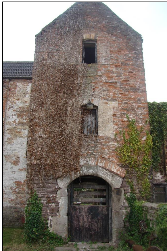
Figure 23: Entrance to the barn (Source: author).
