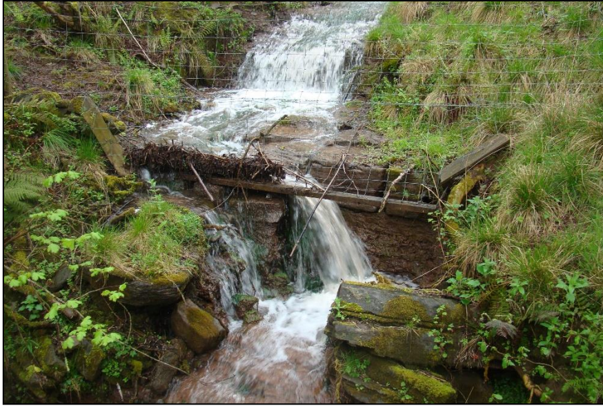
Figure 25: A ford constructed of large slabs of sandstone as the Old Roadway crosses a stream below Ty Isaf farmstead (Source: author).
