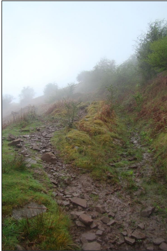
Figure 12; Remnants of an engineered causeway and ditch track from Troed y rhiw gou farm to the Fwddog ridge (Source: author).
