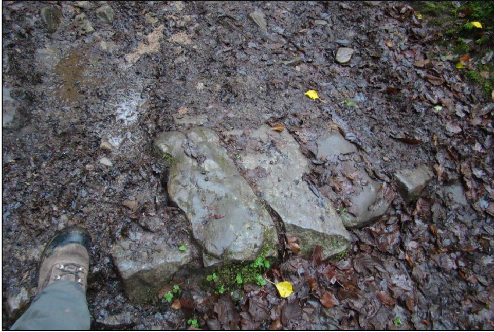
Figure 6: Stone blocks across the track (Source: author).
