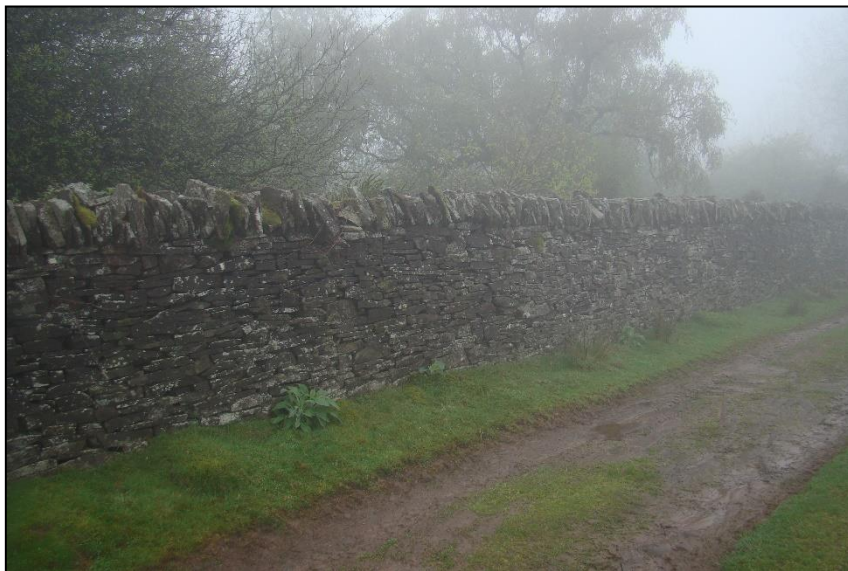
Figure 13: Well-constructed boundary wall on the Fwddog ridge, not simply a field boundary but part of the 'Mountain Wall' that separates the unenclosed upland common grazing land from the fields below. In this case the wall also represents a
