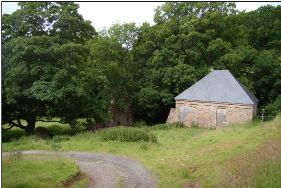
Figure 7: Ruin of The Grove mansion, little remaining of the main house to the left, recently roofed and stabilised coach house to the right (Source: author).
