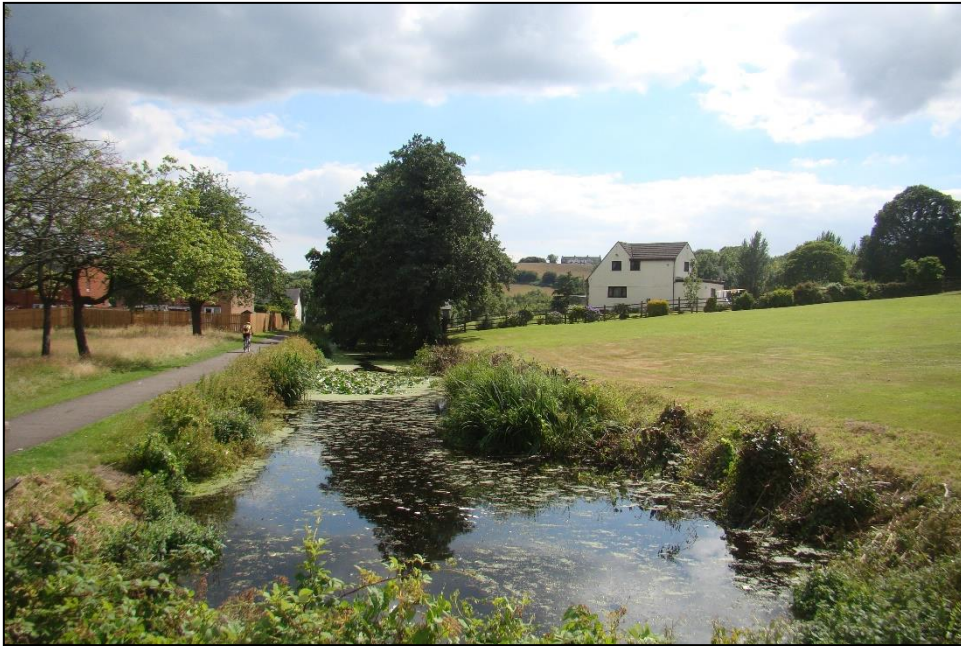
Figure 22: The Pontypool to Newport canal looking southwards (Source: author).
