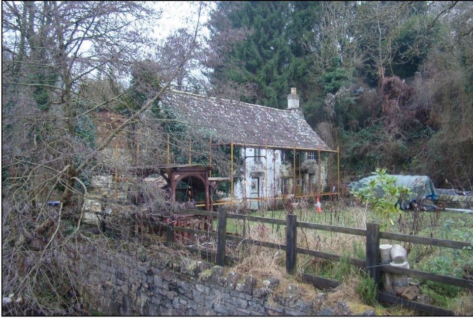
Figure 28: Stankhouse farm under renovation (Source: author).
