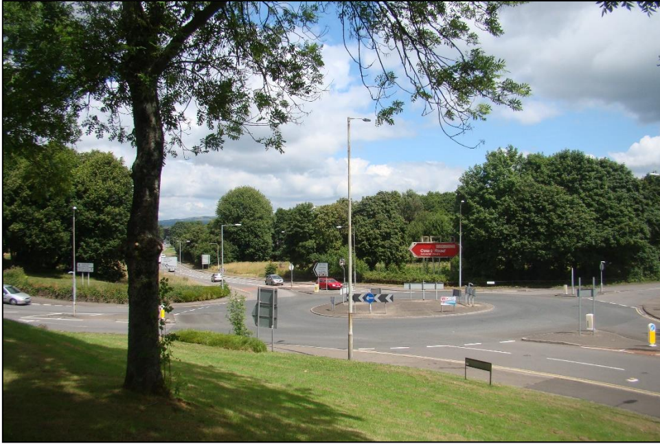
Figure 4: New town roundabout looking north with entrance to Court Road Industrial Estate to right (Source: author).
