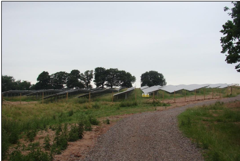
Figure 11: Solar panels on the site of Park Wood (Source: author).
