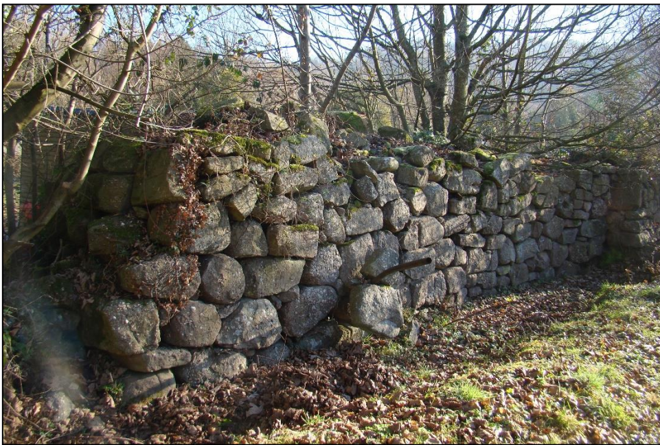
Figure 17: Boulder stone wall, characteristic of the small fields and lanes of the landscape around Brockweir and Hewelsfield (Source: author).
