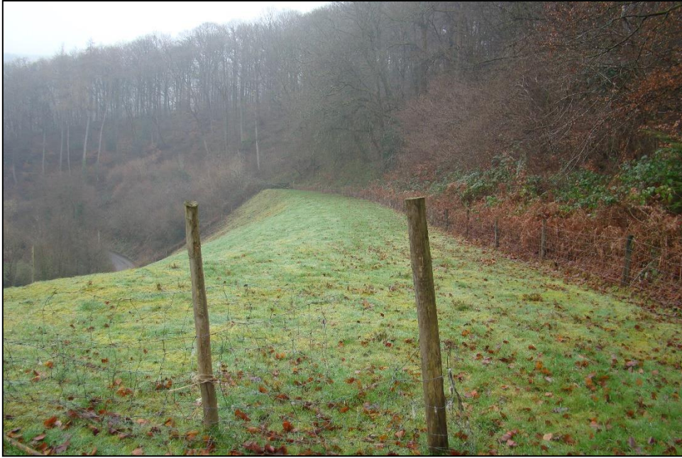
Figure 18: Embankment and surface of a possible tramway above Pont-y-saison (Source: author).
