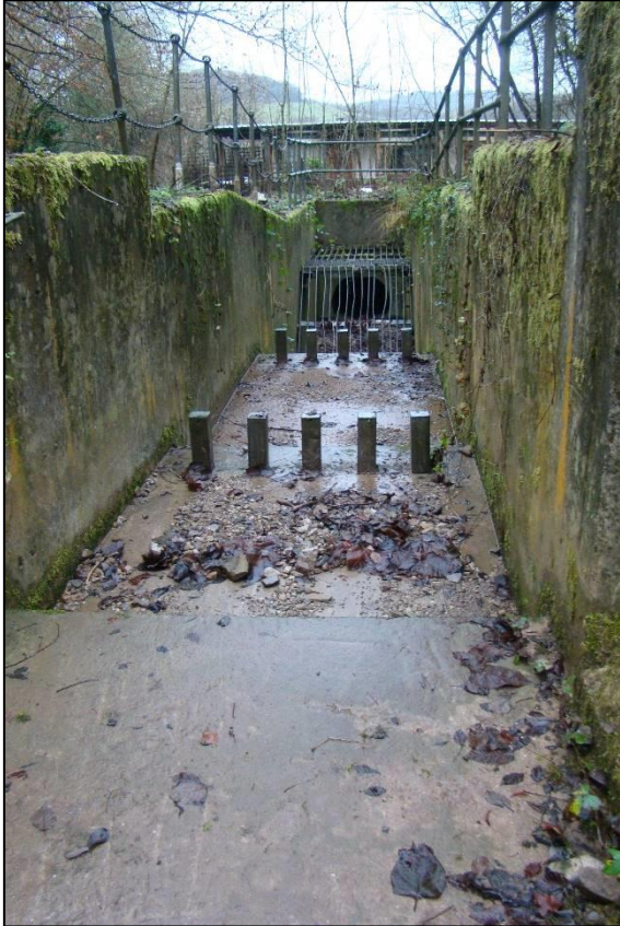
Figure 3: Culvert (Source: author).
