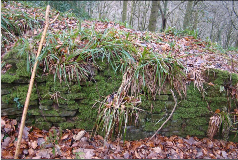
Figure 25: Revetment wall of tracks to Fair Oak (Source: author).
