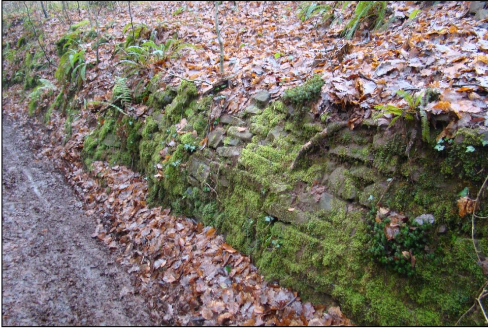
Figure 14: Revetment wall of the track (Source: author).
