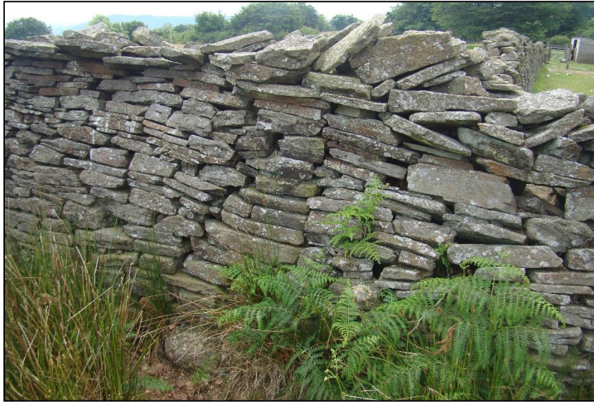
Figure 32: Outer wall of grange land, with quartz boulder visible at base (Source: author).
