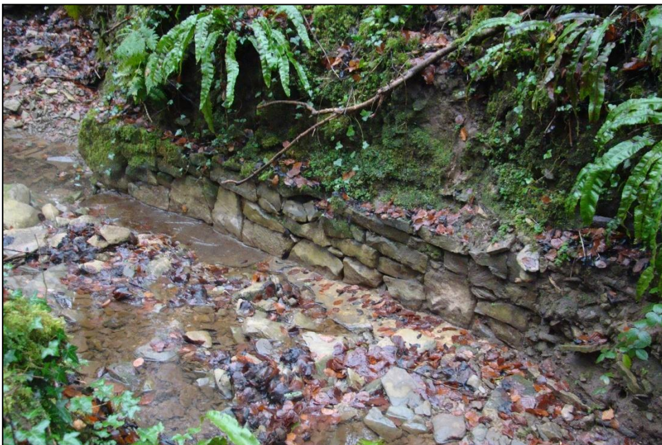
Figure 5: Revetment wall of stream alongside track (Source: author).
