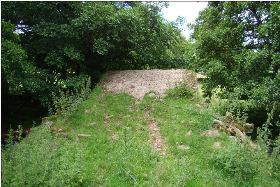
Figures 23 and 24: Landor's bridge at Henllan (Source: author).
