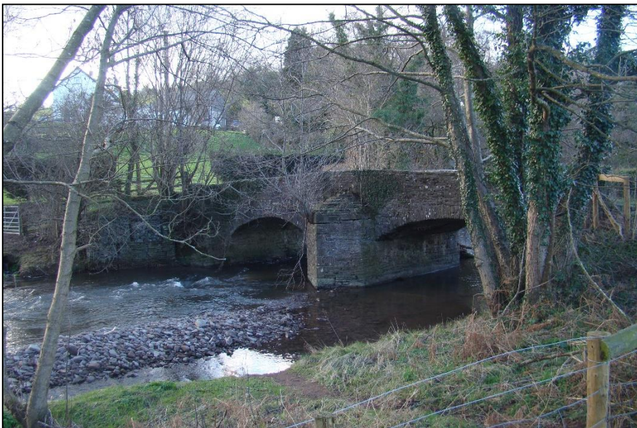
Figure 27: Pont Rees Powell bridge: the start and end of the Cwmyoy boundary survey of 1612 and a key medieval communication and manorial boundary landmark (Source: author).
