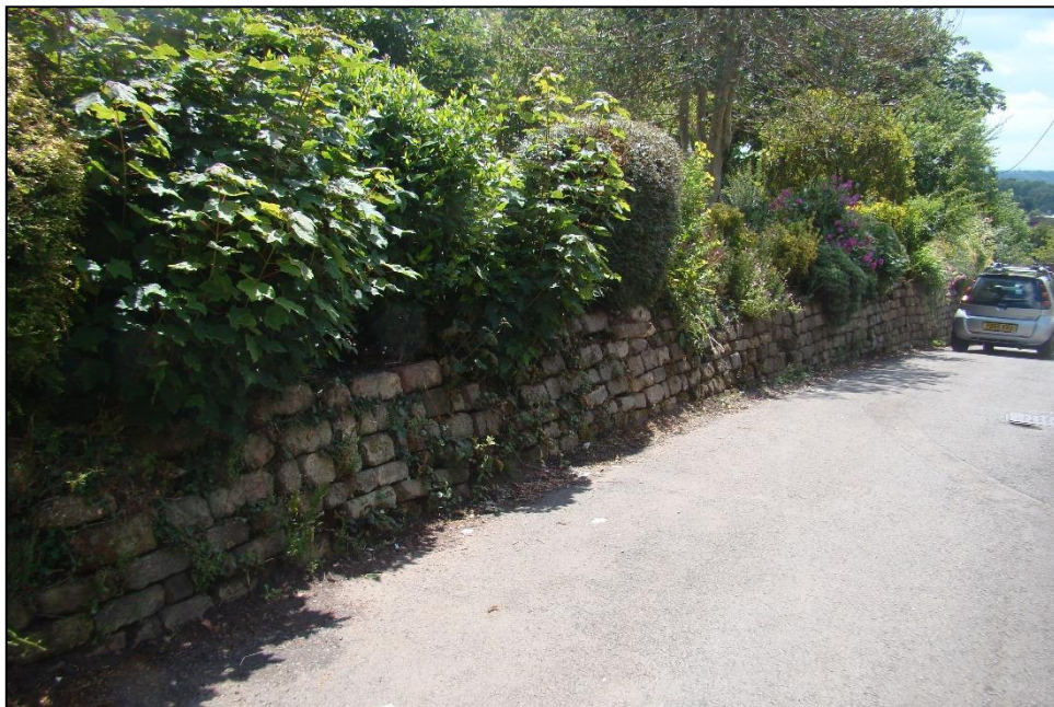
Figure 7: Section of old wall on lane up to St. Dial's (Source: author).
