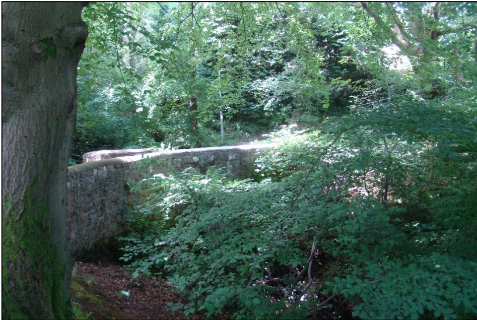
Figure 16: Bridge carrying the lane, hidden away behind the suburban closes (Source: author).
