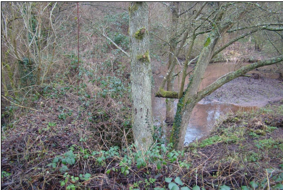
Figure 19: Pond and dam of the Upper Forge (Source: author).
