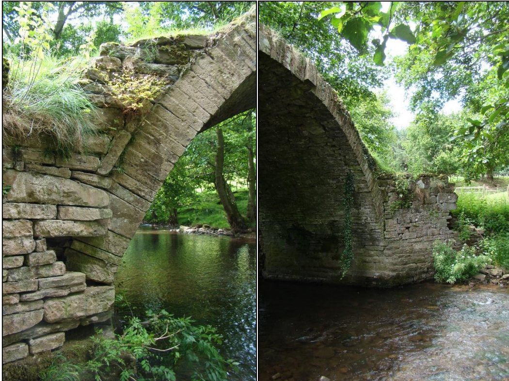
Figures 20, 21 and 22: Landor's bridge at Henllan (Source: author).
