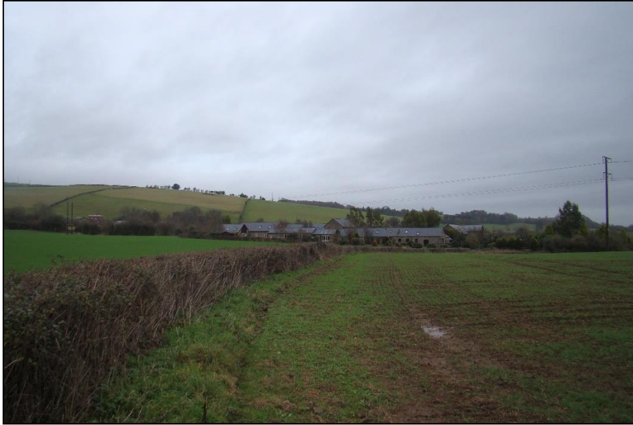
Figure 30: Rogerstone Grange, looking north (Source: author).
