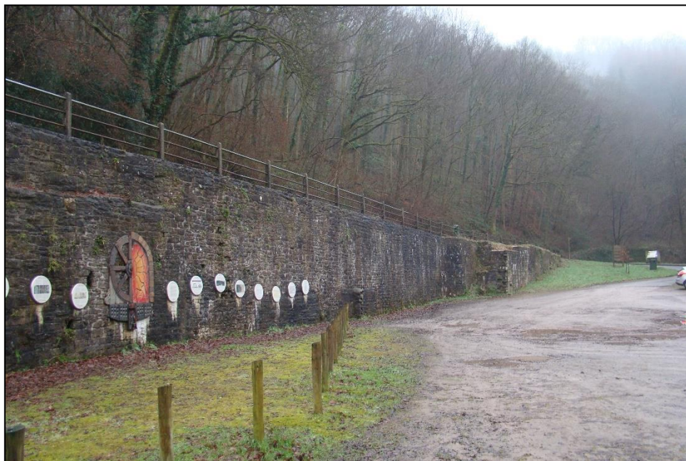
Figure 1: Site of the Lower Wire Works, Angidy Valley (Source: author).
