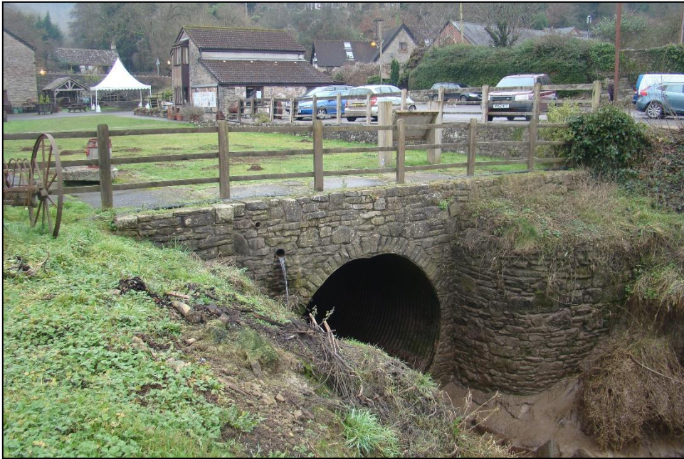
Figure 26: The filled in tidal dock at the mouth of the Andigy Brook (Source: author).
