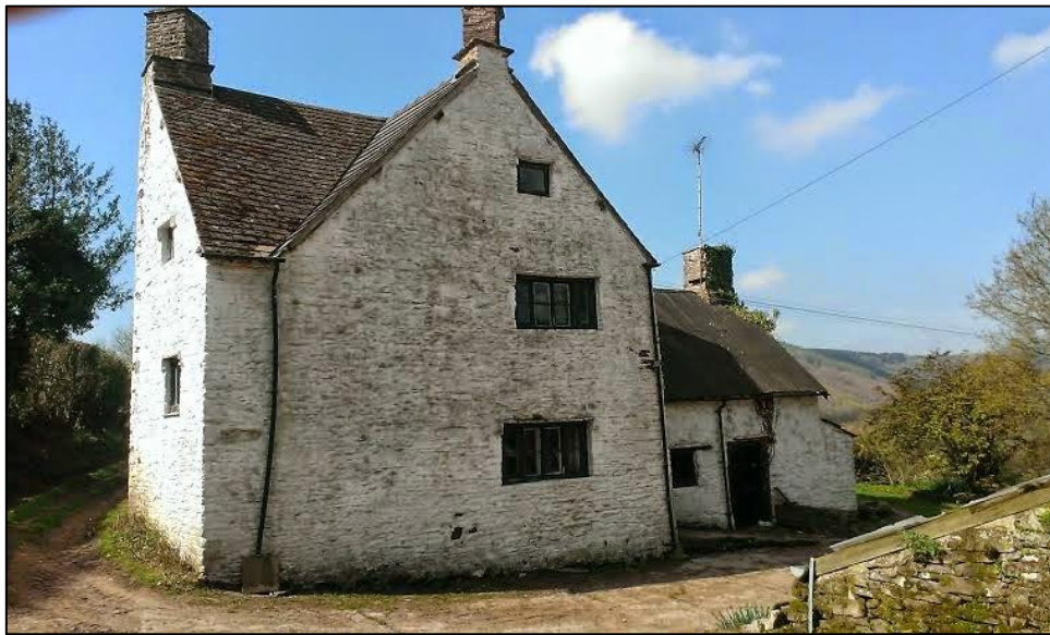
Figure 5.23: Eastern elevation of Little Lwygy, with the Tudor period portion of the house to the right (Source: author).
