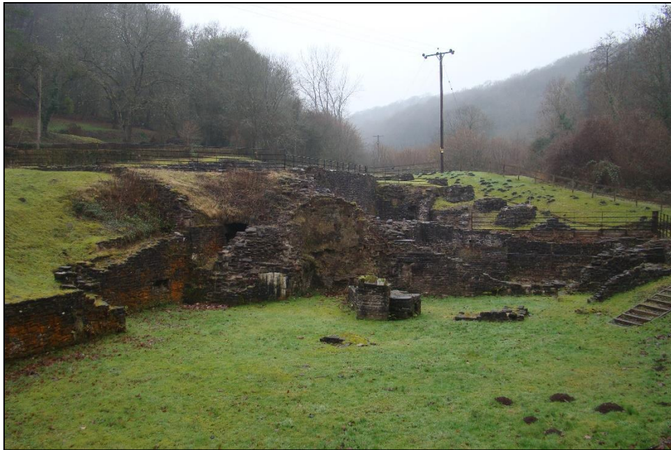
Figure 8.22: The remains of Abbey Tintern Furnace above the abbey in the Angidy Valley (Source: author).
