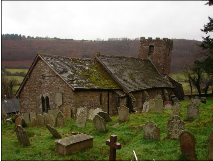
Figure 5.34: The eastern elevation of St. Martin's church, Cwmyoy (Source: author).
