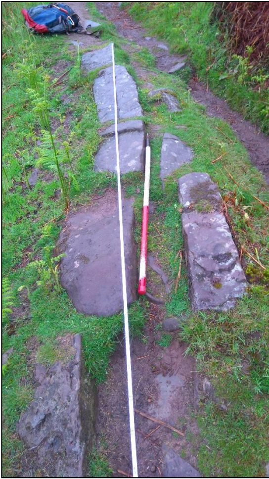
Figure 11.11: Part of the constructed Fish Path at Cwm-bwchel above Llanthony (Source: author).
