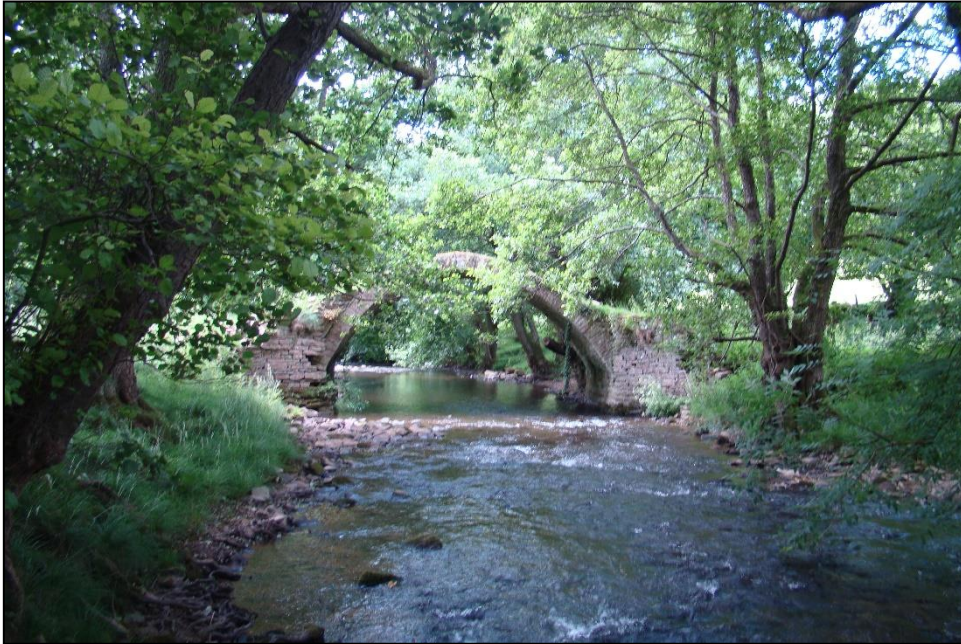
Figure 6.27: Landor's ruined bridge at Henllan (Source: author).
