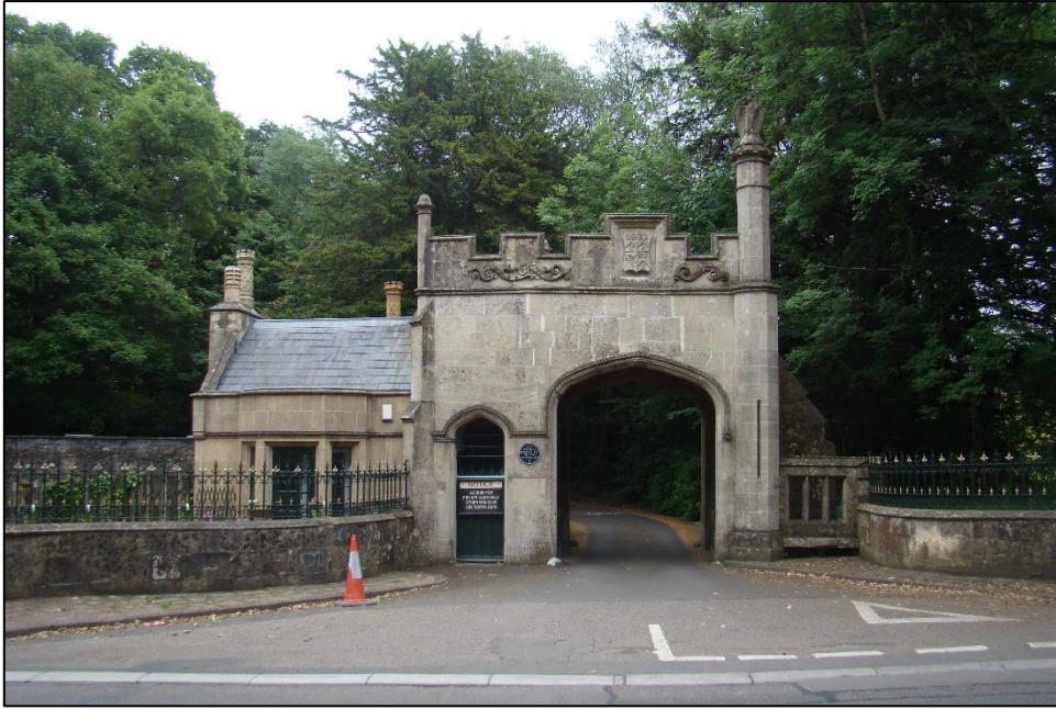
Figure 10.11: The new and repositioned 'Magna Porta' gatehouse of 1836, through which the new driveway met the straightened Turnpike road (Source: author).
