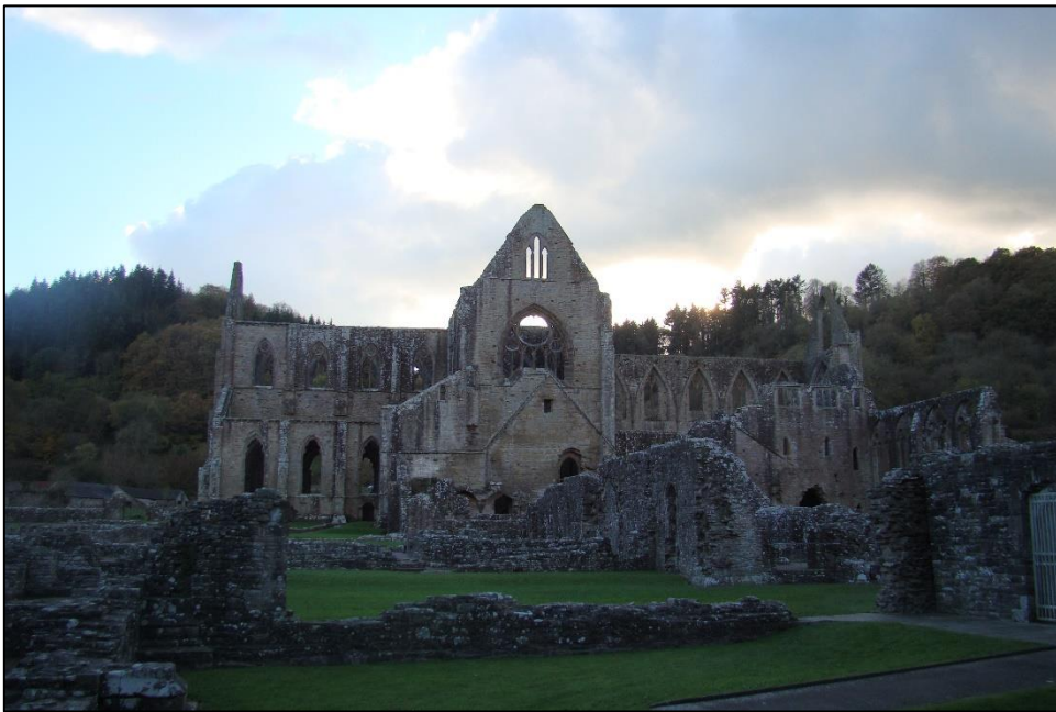
Figure 4.5: Tintern’s abbey church and the remains of other claustral buildings, looking west (Source: author).
