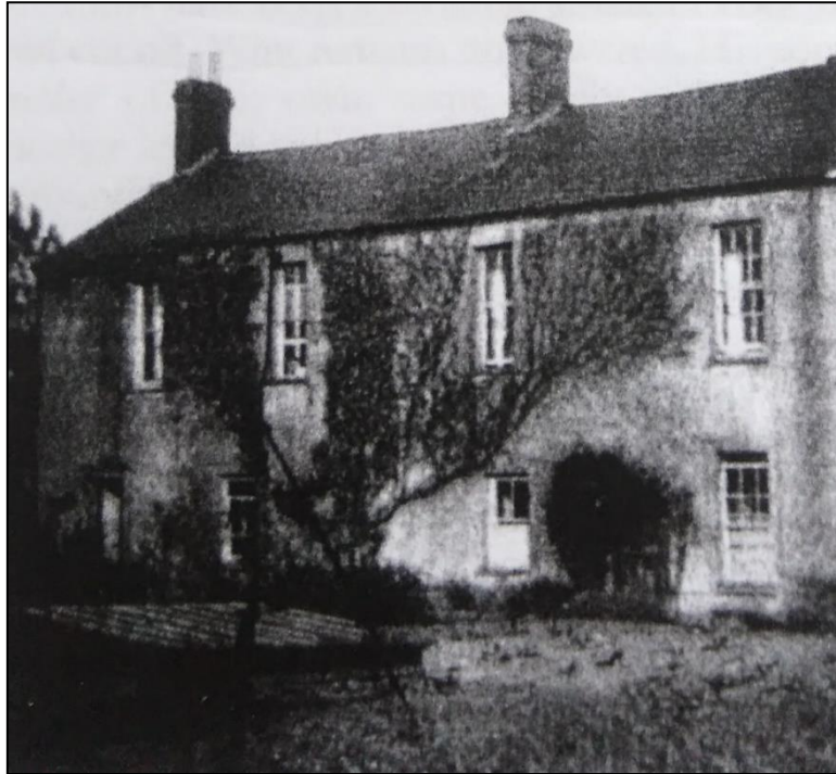
Figure 9.22: A rare image of Court Farm circa 1950 a few years before its demolition (Source: after John 2007, 130).
