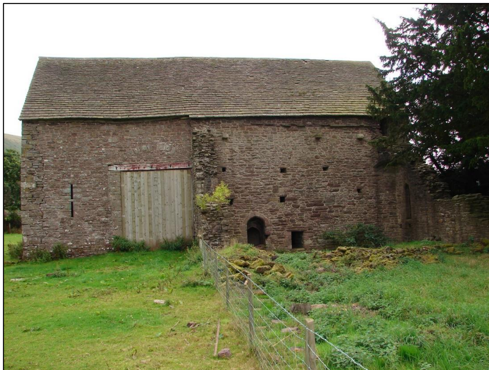
Figure 5.19: The northern elevation of the fourteenth century gatehouse at Llanthony, with post-medieval barn extension to the left (Source: author).
