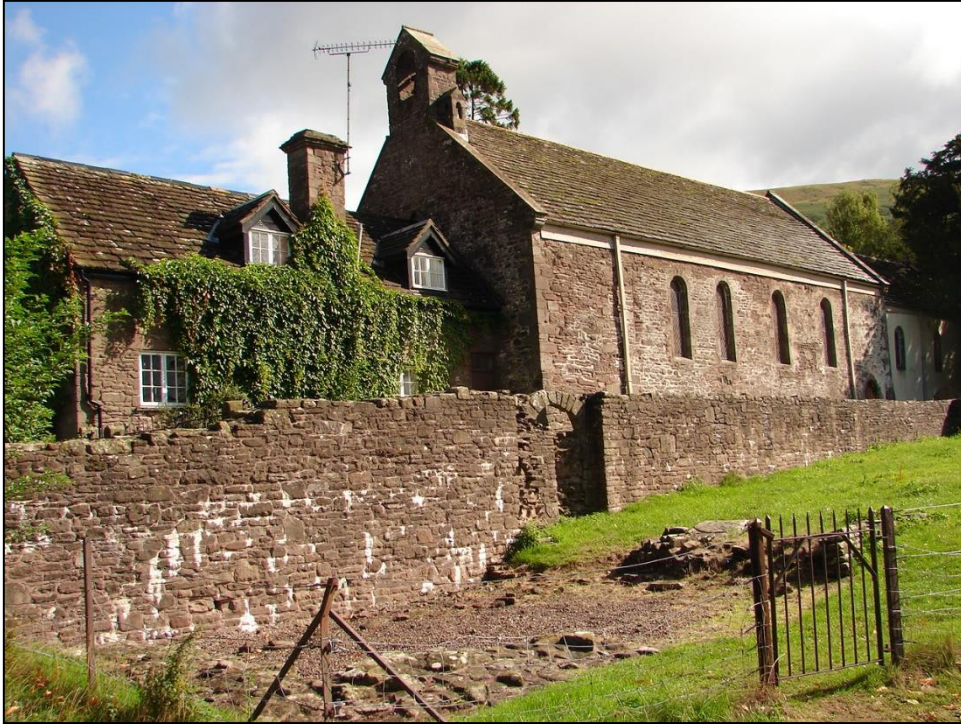
Figure 6.7: St. David's parish church occupying the site of the priory infirmary (Source: author).
