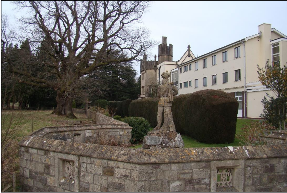
Figure 10.39: Modern extension to the nineteenth century Llantarnam Abbey house (Source: author).
