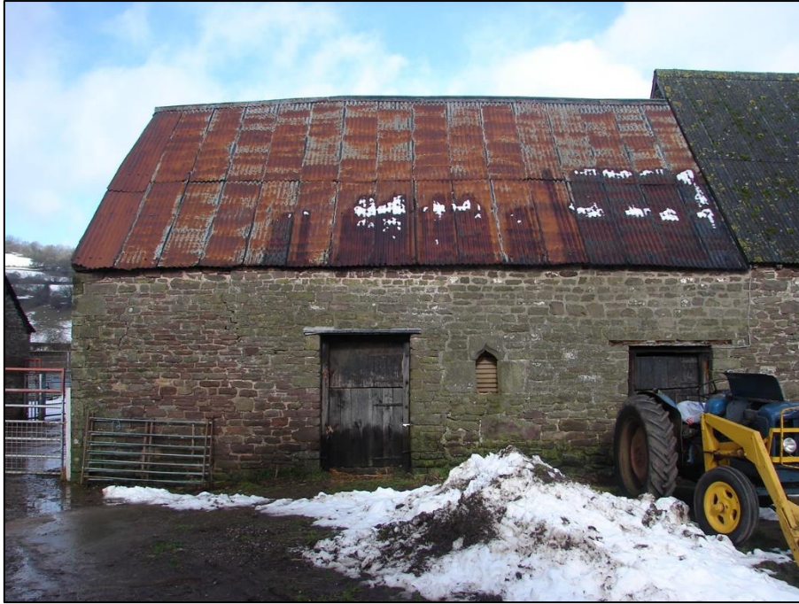
Figure 5.36: The southern elevation of the priory chapel for Stanton manor with ogee-headed lancet window clearly visible (Source: author).
