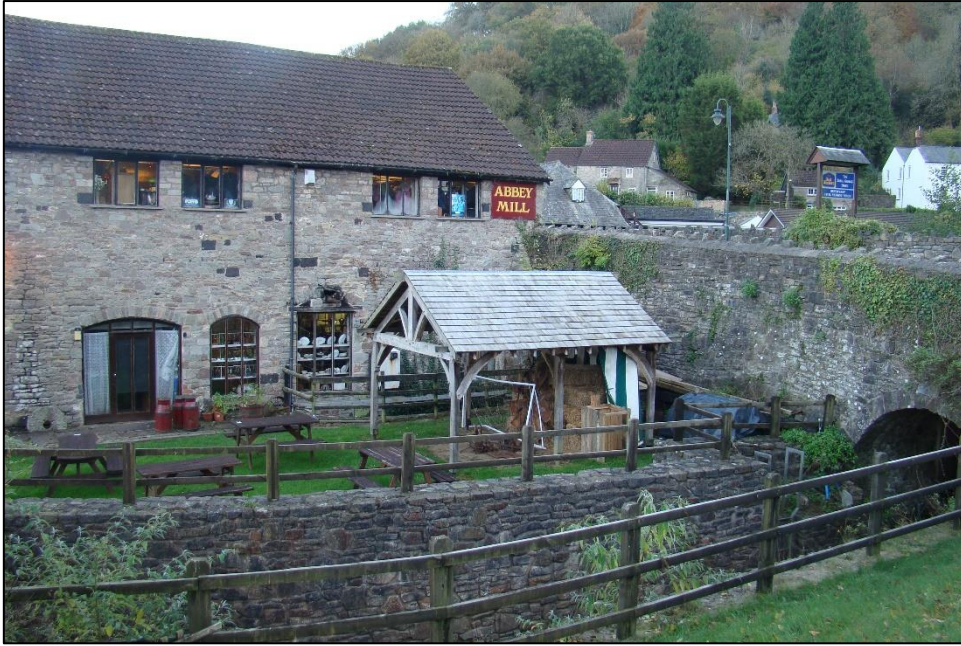
Figure: 7.50: The post-medieval Abbey Mill alongside the Angidy Brook on the northern limit of the precinct, likely site of the original monastic mill (Source: author).
