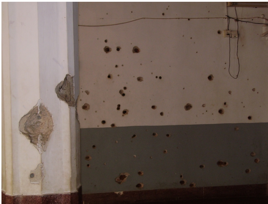
Figure 6: The bullet holes are still present in the mosque and maintained as a reminder (picture taken by the author on a visit to the mosque in March 2006)
