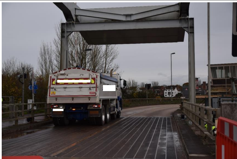
Figure 4.34 Picture for truck load test on the bridge (LP4).
