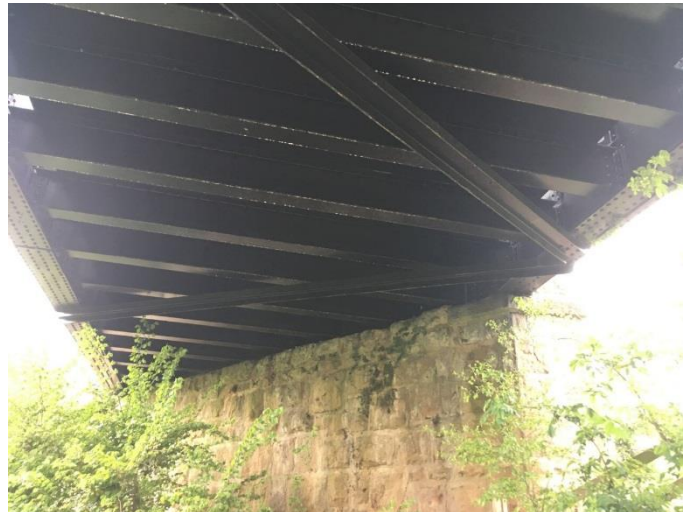
Figure 5.3 Superstructure of Mineral Line Bridge.
