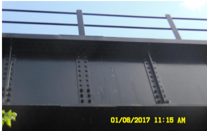
Figure 5.5 Transverse intermediate stiffeners riveted to web girder.
