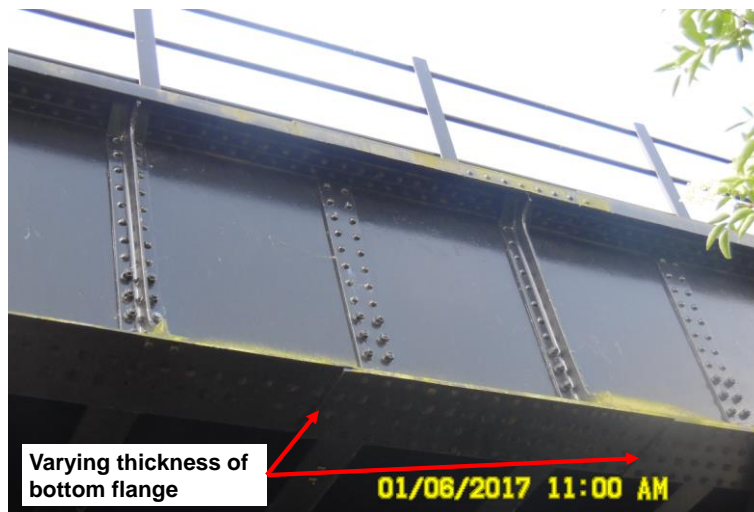
Figure 5.4 The varying thickness of bottom flanges of the main girder.
