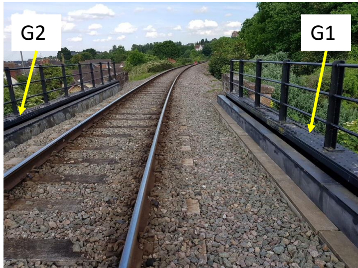
Figure 5.14 Photo of the track system of the Mineral Line Bridge.
