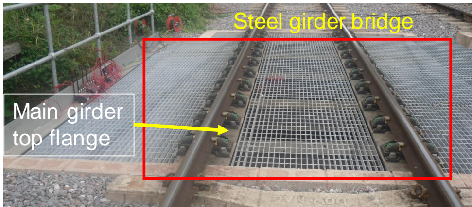
Figure 5.41 Photo of the track -line shown the Williton Up Bridge.
