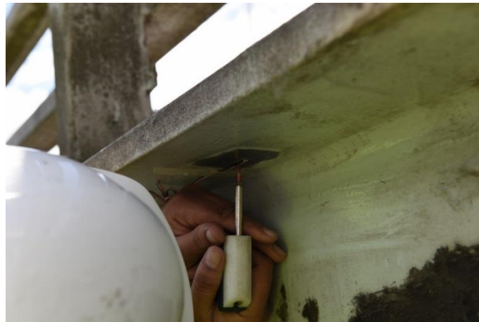
Figure 4.15 Picture of a weldable strain gauge being installed on the bridge.
