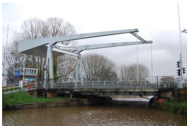
Figure 4.2 The Bascule Bridge.
