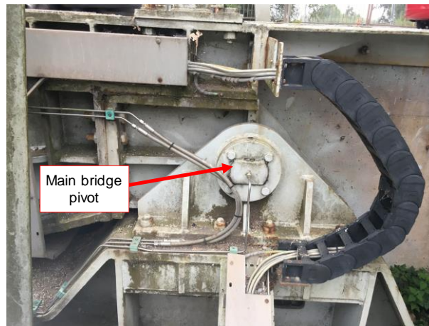
Figure 4.11 The pin support of the bridge.
