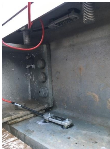
Figure 5.46 Photo showing typical installation of BDI sensors at mid span.
