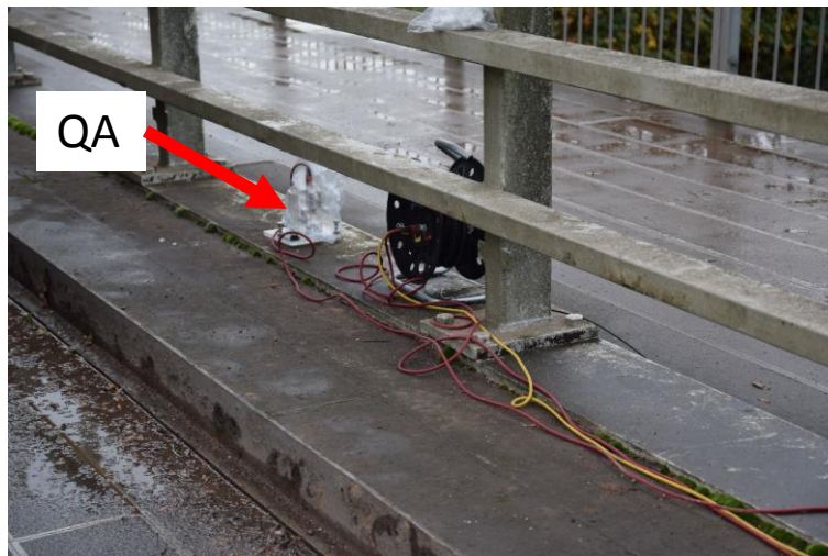
Figure 4.23 QA in use during a load test.
