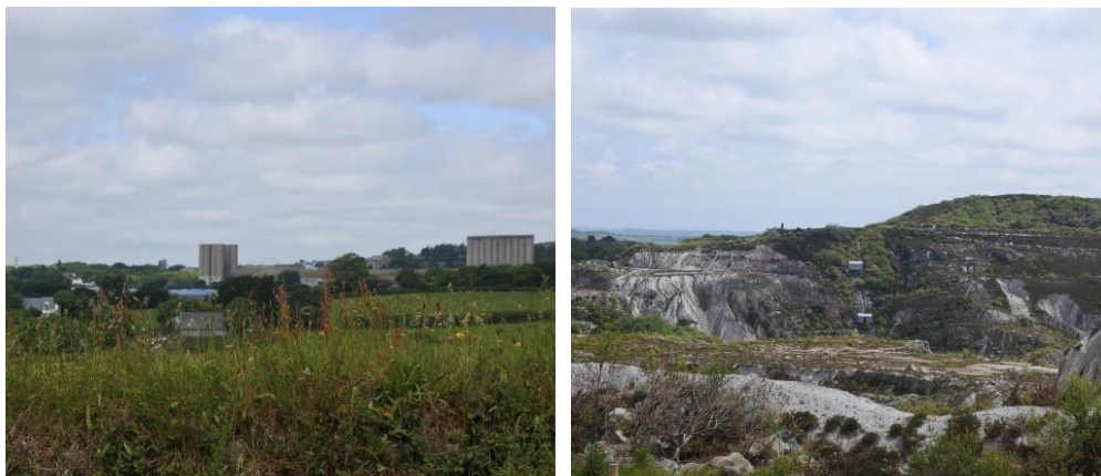
Figure 5.2 (left) Concrete towers of the Blackpool dries rise into the sky over the village of Trewoon. Photo by Author
