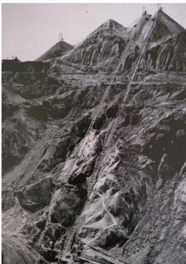
Figure 3.10 (left) Double incline railway and tips at Dubbers china clay works. Photo © Rita Barton 1966
