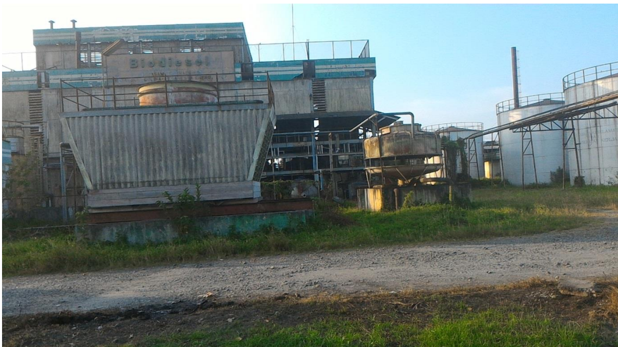
Picture 5.3 Abandoned Biodiesel Facilities
