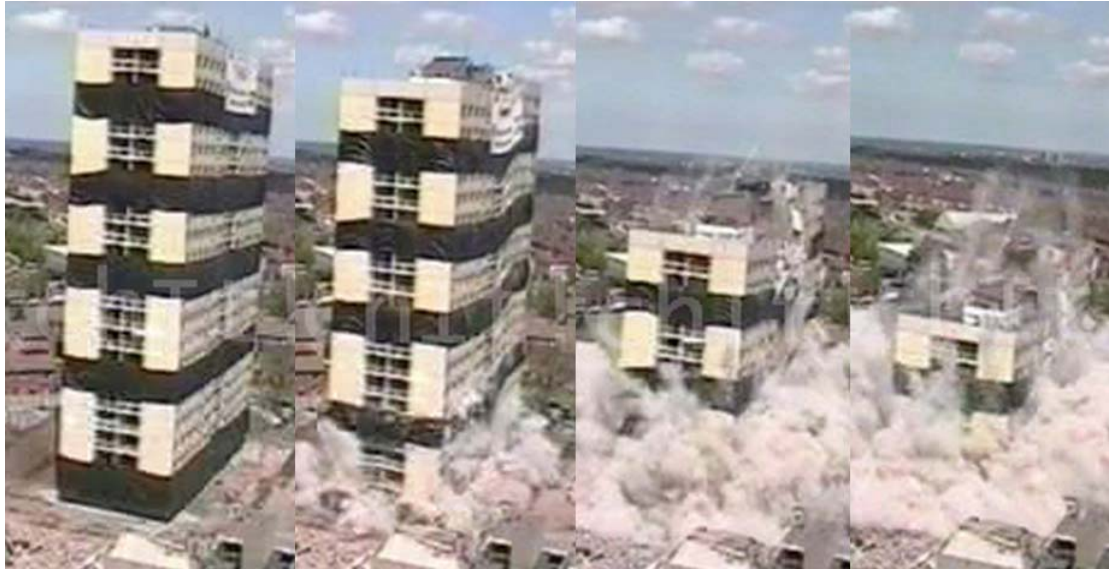
Figure 1. Implosion of Kenley Tower.
