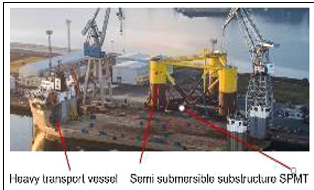
Figure 3. Semi sub. loadout from land. 7
