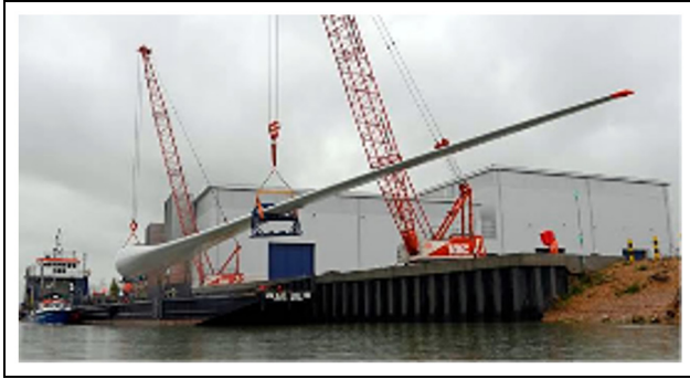
Figure 7. Blade loadout from quay. 17
