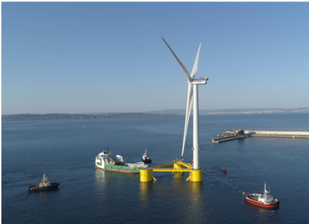
Figure 3 Steel Semisubmersible under tow ref. [ https://www.principlepower.com ]
