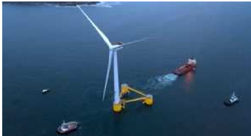
Figure 5 Semi submersible with turbine tow out (courtesy Principle Power)
