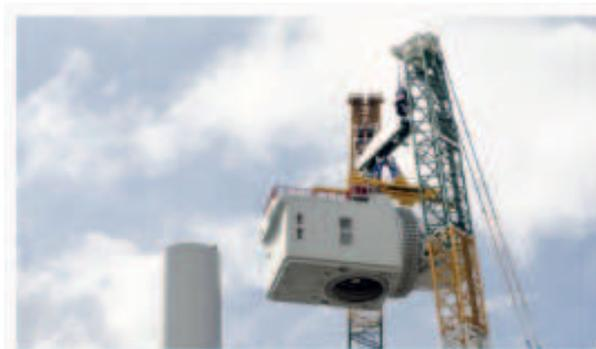
Figure 9 Nacelle lifting [5]
