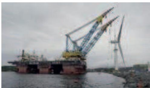
Figure 6 Spar topsides lift off quay
