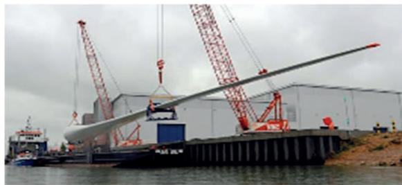
Figure. 7 Blade load out [16]
