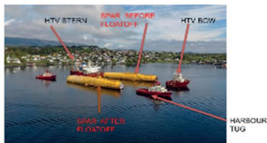
Figure 5 Spar float off before upending [14]
