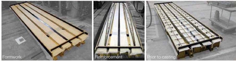
(a) Steps of the construction process of steel-reinforced shape optimised concrete beams (Orr (2012))
