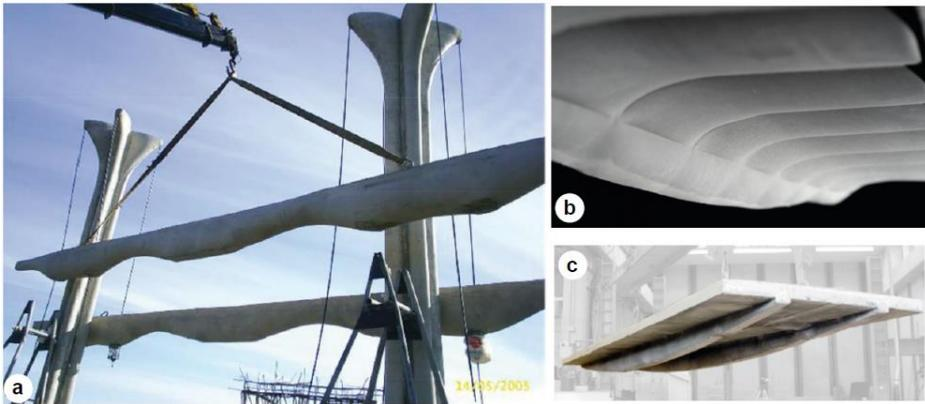
Fig. 1 Shape-optimised reinforced concrete beams cast using flexible fabric formwork (Hawkins et al. [3] for (a) and Orr [4] for (b) and (c))
