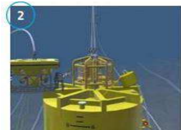
Figure 13 Suction pile installation(credit Acteon)
