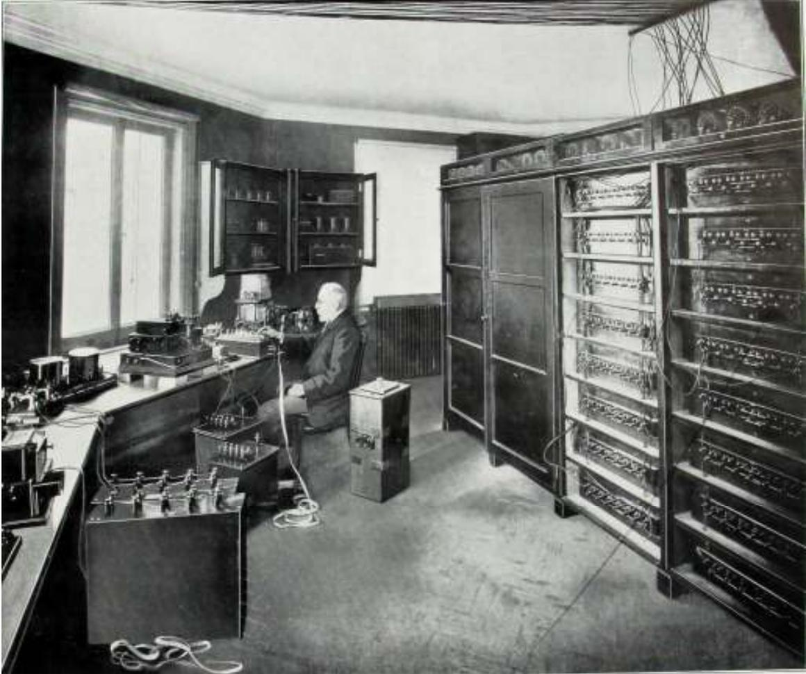
FIGURE 3: The Electra House laboratory in 1902. Here the Electrician-in-Chief Henry Saunders is seen testing the performance of a siphon recorder whose paper tape trails onto the floor. Behind him looms a large cabinet housing the ‘artificial line’: Anon., ‘Electra House: the New Home of the Eastern and Associated Telegraph Companies’, *Builder’s Journal and Architectural Record*, 20 August 1902, pp. 1-13, p. 10 (Image courtesy of Porthcurno Telegraph Museum).
